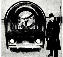
Constructed as a demonstration model for government officials this strange automobile pictured here with its inventor, Thomas Finley, is driven by a propellor revolving in a wind tunnel.
